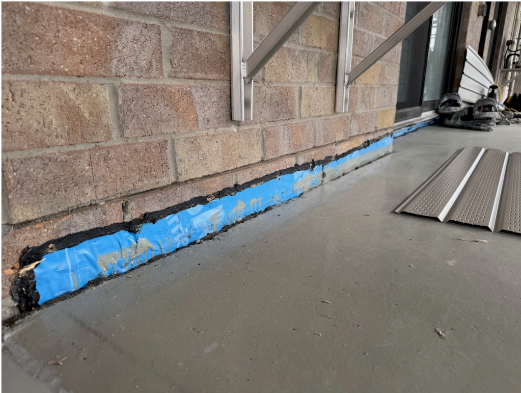
Photo 5: Blueskin membrane sealed the leading edge to the brick cladding.
