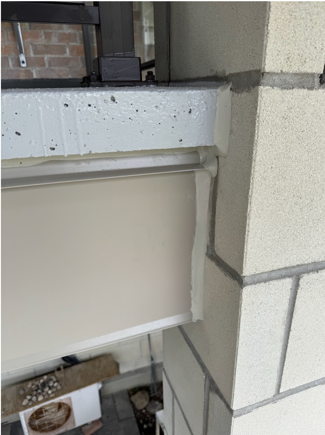
Photo 25: Close-up of the completed caulking.
