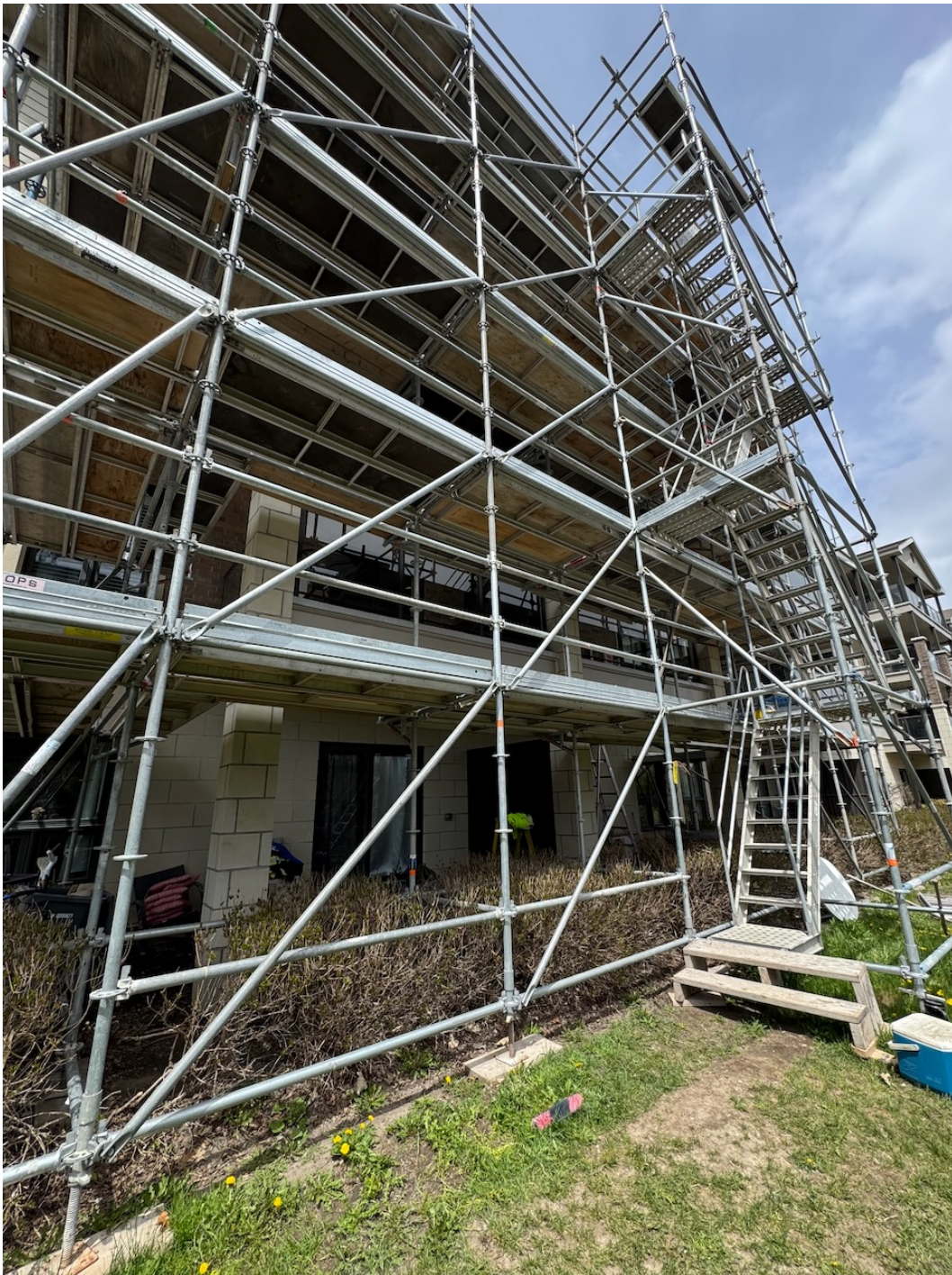
Photo 20: Drop 14 - May 11 - General view of the completed drop.
