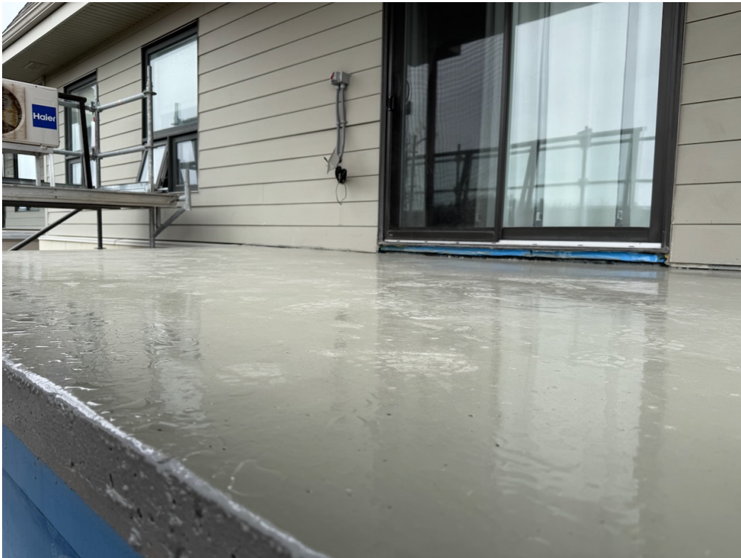
Photo 19: Traffic topping base coat complete.
