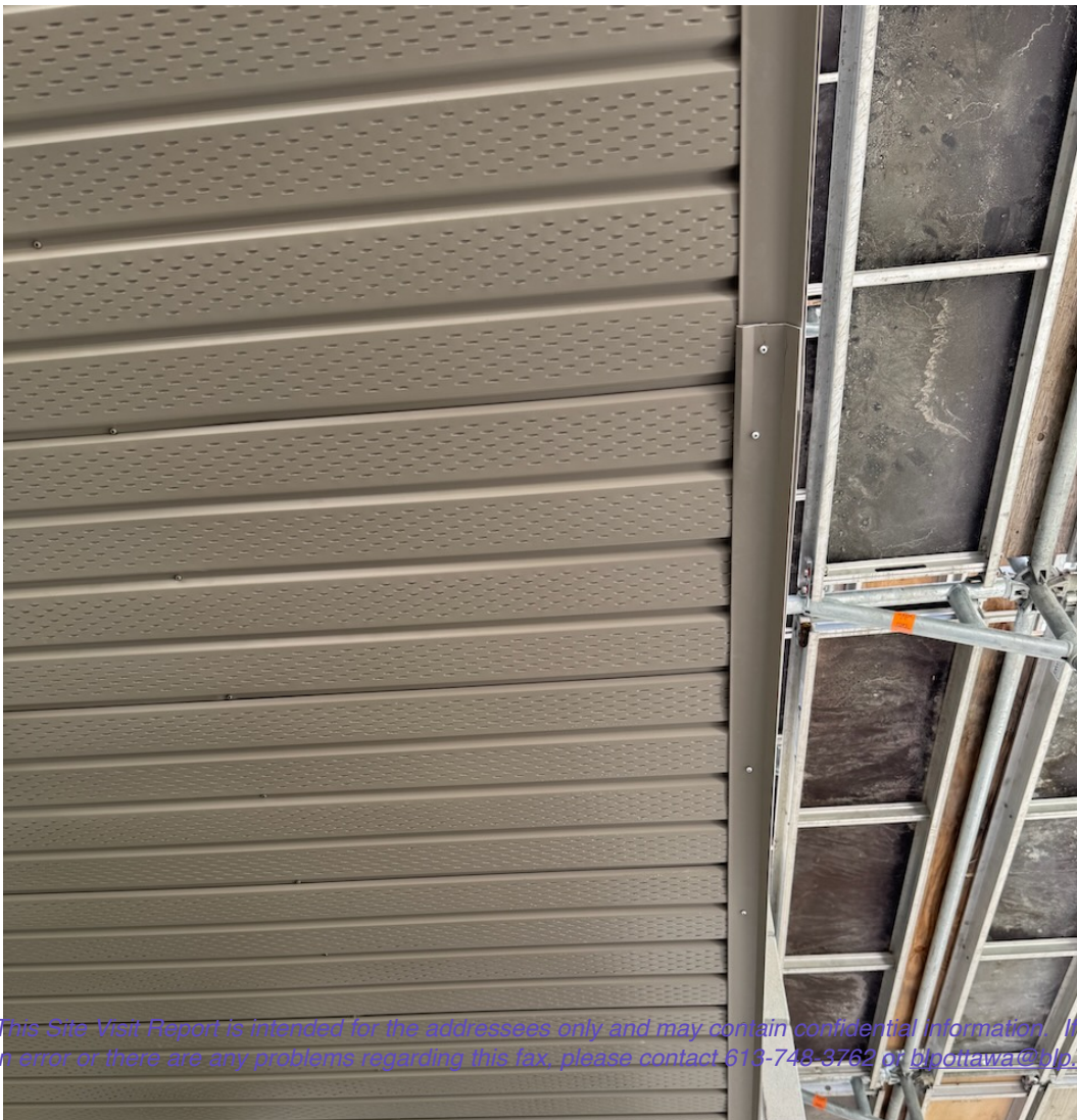
Photo 21: Soffits, flashing, and lights complete. These lights were replaced with new, as close as possible match to the original.
