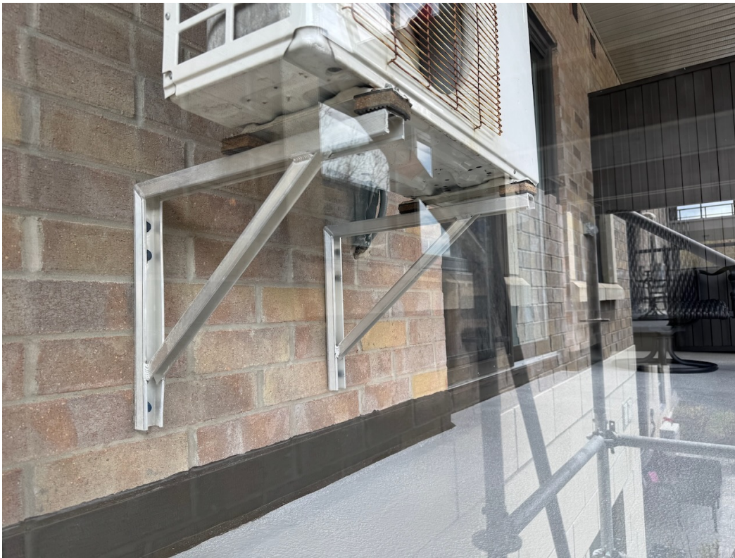
Photo 29: Base wall flashing and caulking complete. A/C unit re-installed.
