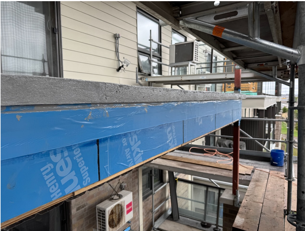
Photo 16: Blueskin membrane and traffic topping membrane complete.
