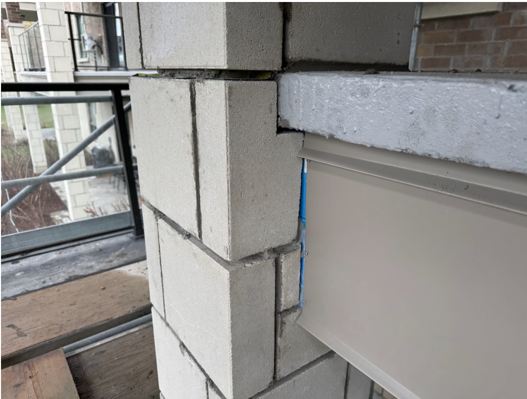
Photo 4: Balcony element installation ongoing.
