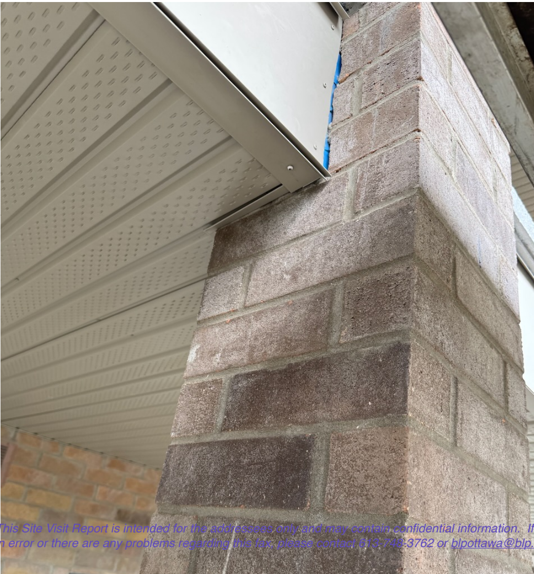
Photo 8: Masonry column cladding complete.
