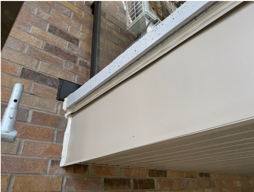
Photo 32: Flashing, caulking, and balcony traffic topping membrane complete. Guardrails re-installed.
