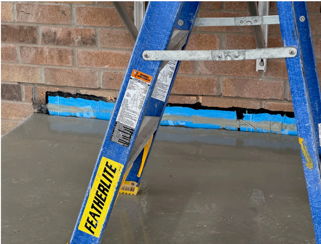
Photo 13: Blueskin membrane sealed the leading edge to the brick cladding.
