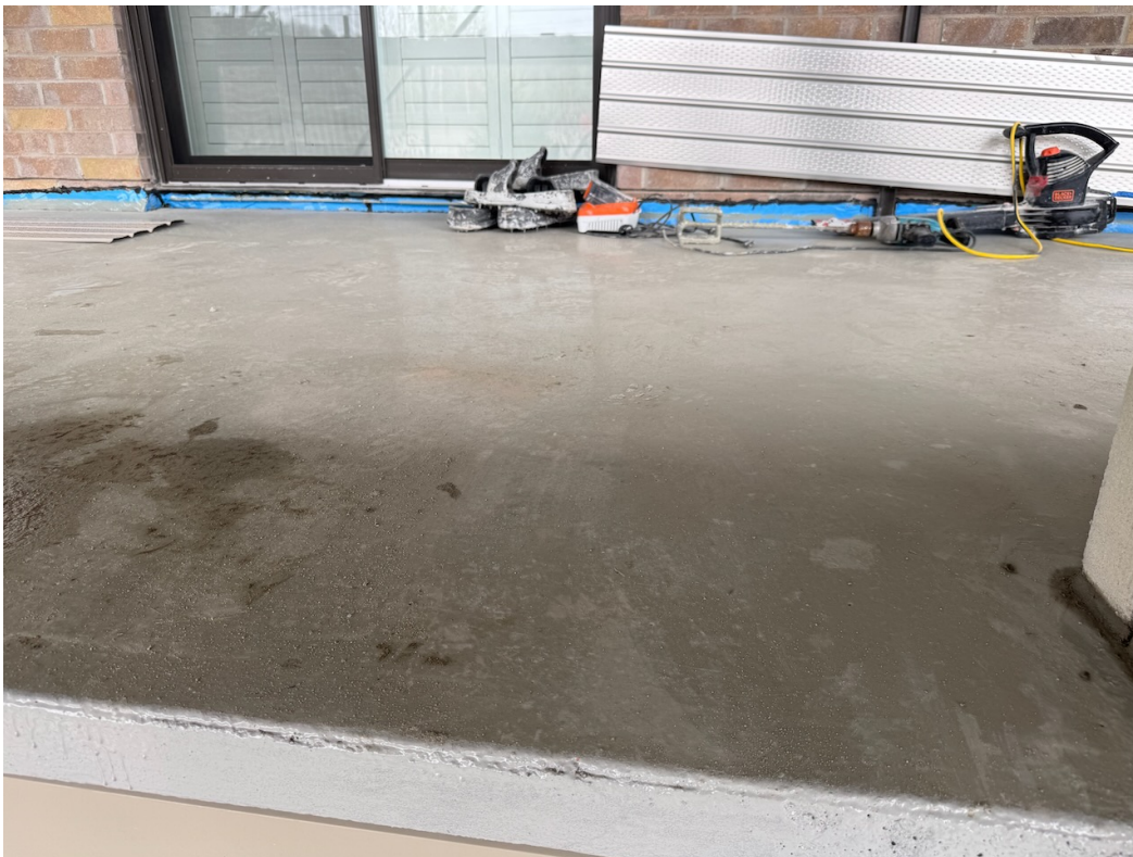
Photo 3: Base coat of the balcony traffic topping membrane.
