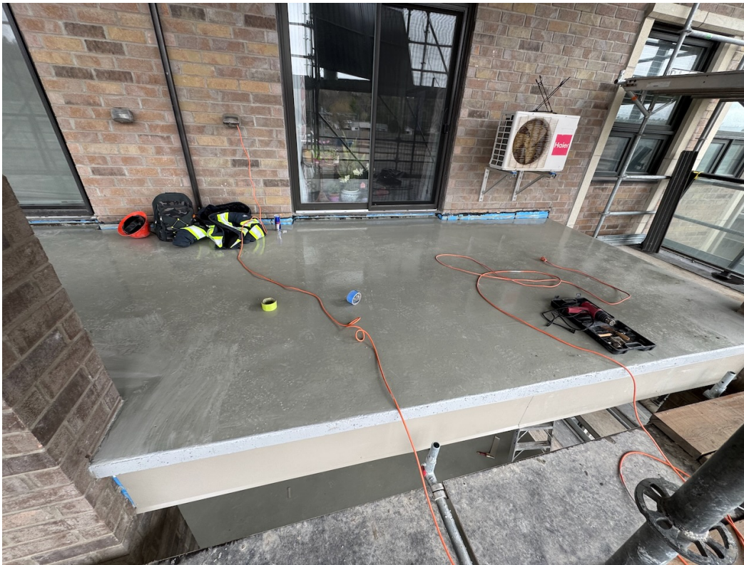
Photo 10: Base coat of the balcony traffic topping membrane.
