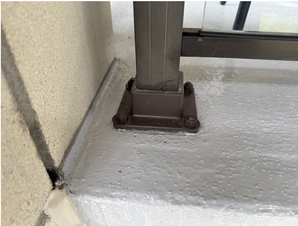
Photo 27: Guardrails re-installed.
