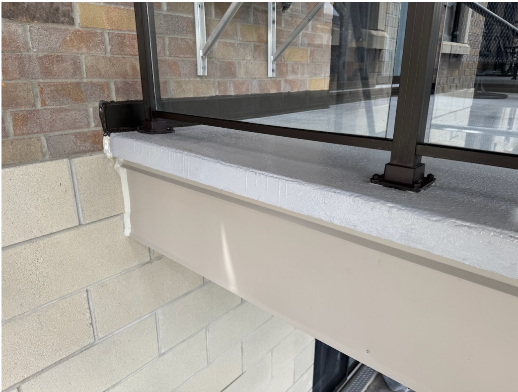
Photo 28: Flashing, caulking, and balcony traffic topping membrane complete. Guardrails re-installed.
