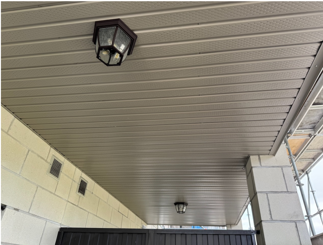
Photo 21: Soffits, flashing, and lights complete. These lights were replaced with new, as close as possible match to the original.
