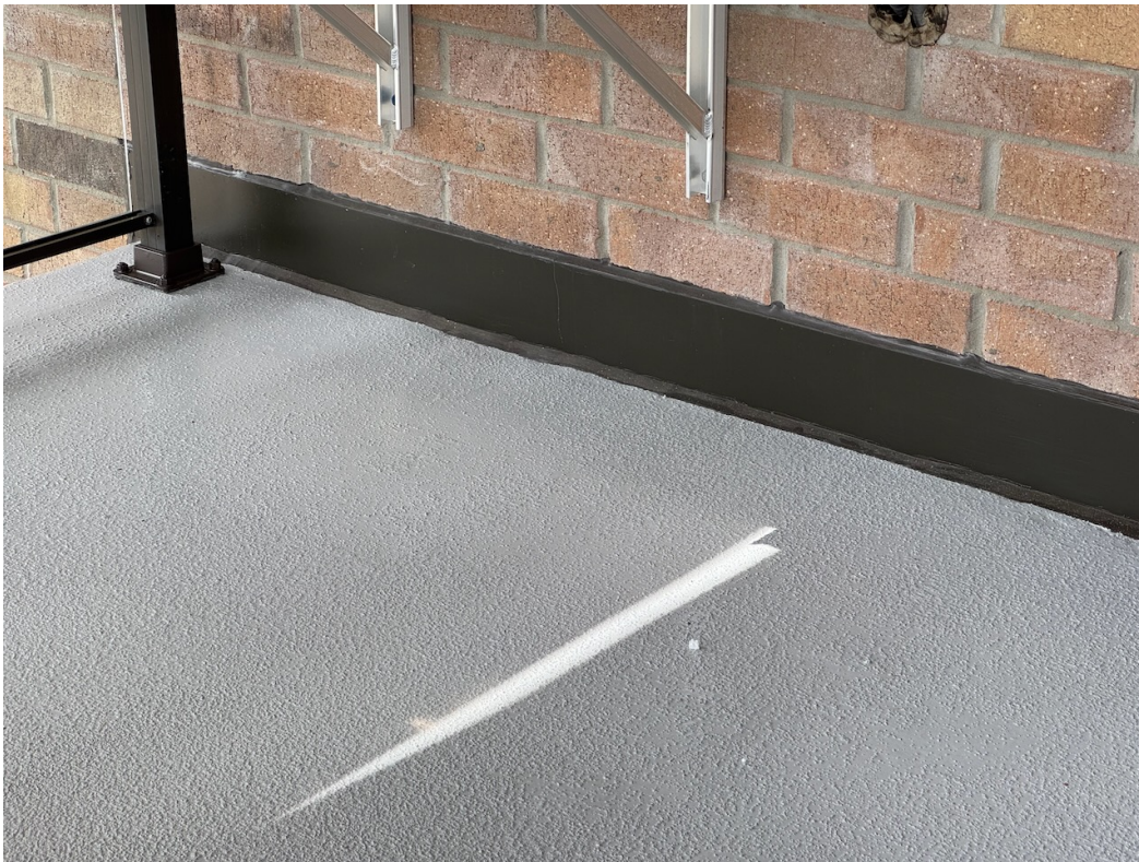
Photo 37: Complete base wall flashing and caulking complete.
