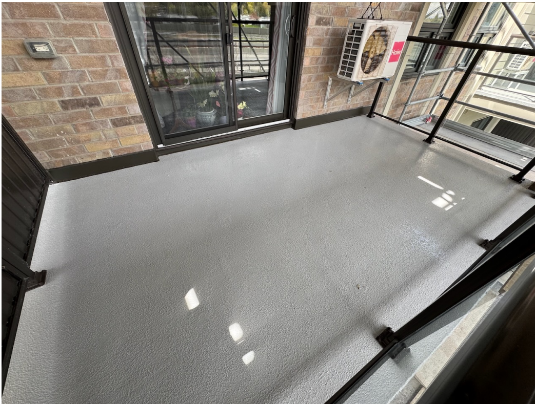
Photo 39: Traffic topping membrane complete.
