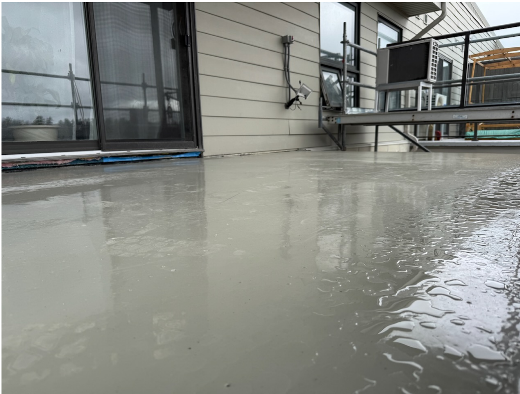
Photo 18: Traffic topping base coat complete.
