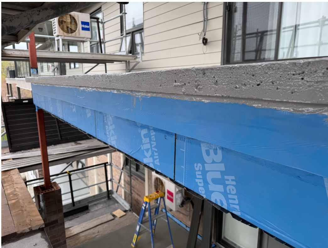
Photo 17: Blueskin membrane and traffic topping membrane complete.
