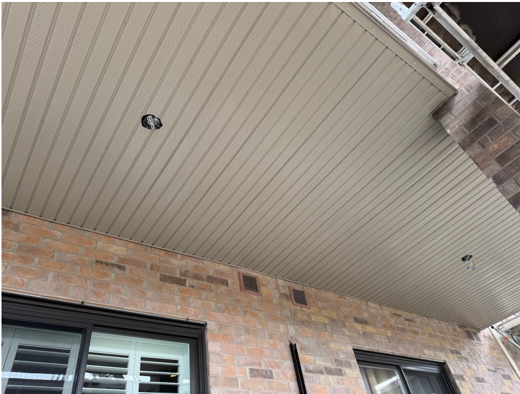
Photo 6: Soffit re-installation complete.
