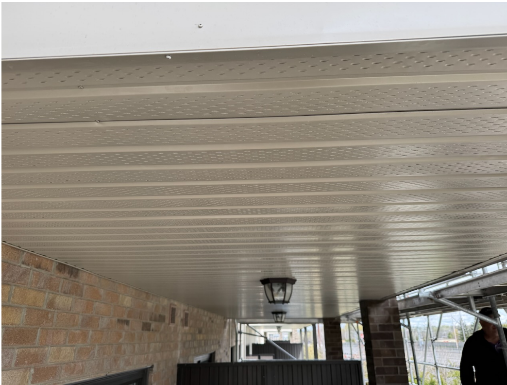
Photo 31: Soffit and light fixtures re-installed.
