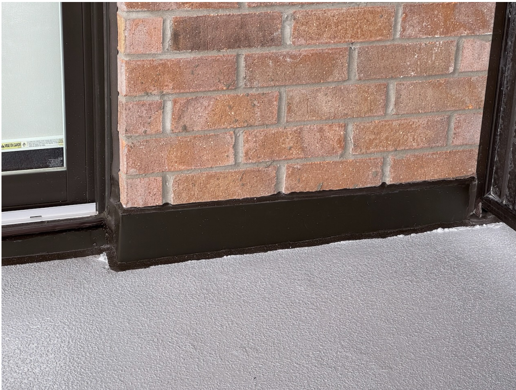
Photo 38: Complete base wall flashing and caulking complete.
