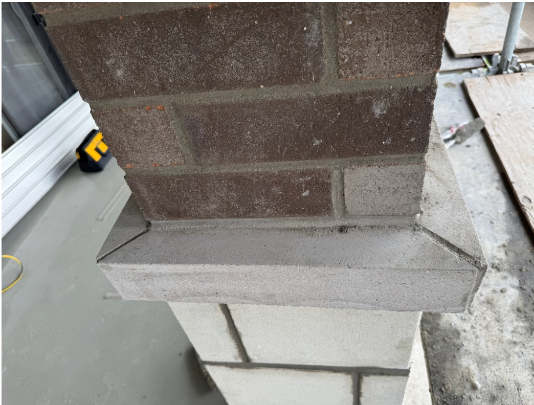
Photo 8: Masonry column cladding complete.
