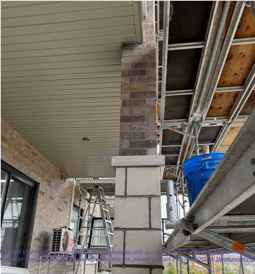
Photo 6: Soffit re-installation complete.
