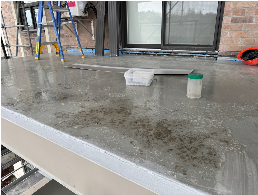
Photo 12: Base coat of the balcony traffic topping membrane.
